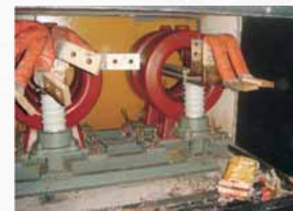
Generator output 6000:1 Test Result
